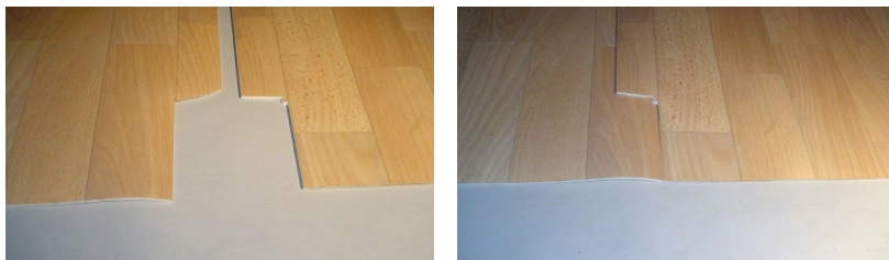
Cutout windows at the seam to align pattern
