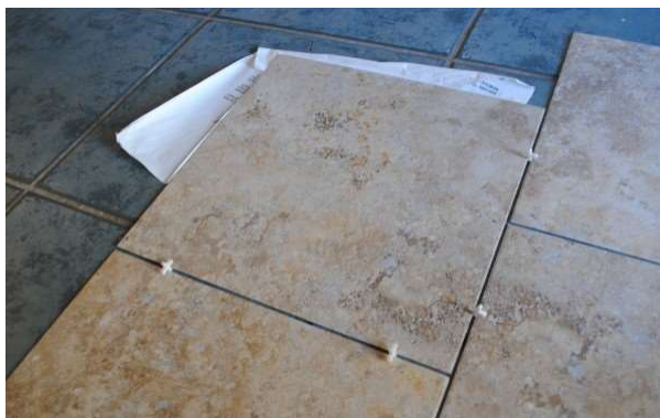
Fig. 1 - Use spacers to maintain the joint width
